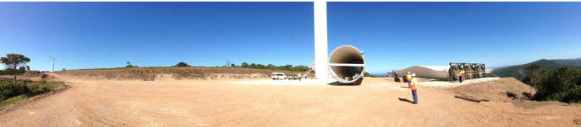
Van Staden's Wind farm, 27 MW – Round 1 project under REIPP
